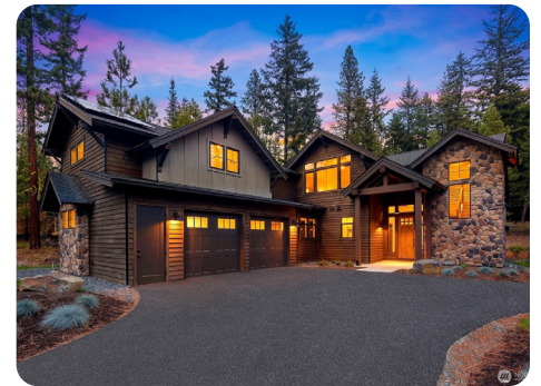
Construction of Luxury Build $1,325,000 | 60% LTV CLE ELUM, WA
