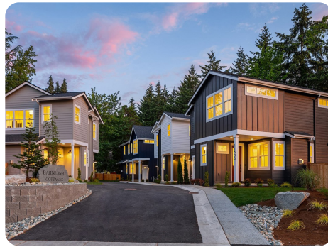
Four Cottage Construction $2,025,000 | 66% LTV KIRKLAND, WA
