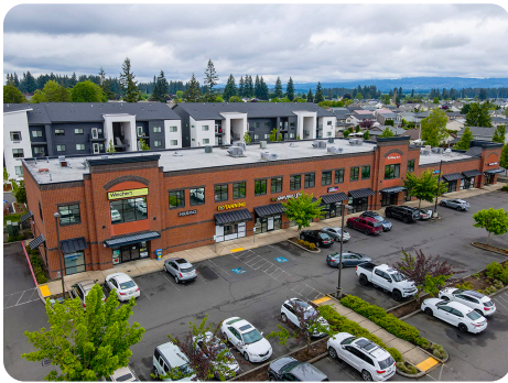
Commercial Refinance $3,100,000 | 59% LTV VANCOUVER, WA
